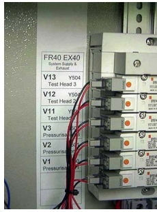
Figure 1.1 50 Million Cycle Valves. An LT2 installation typically has to do over 10 million cycles per year!
